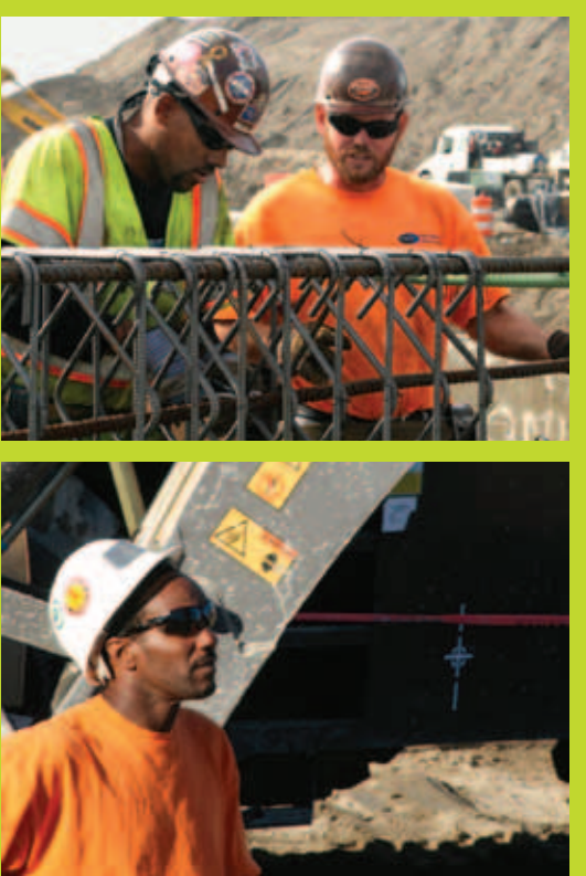
Construction crews at work on the site of The New Wishard.
